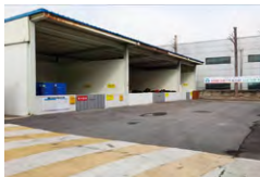
Separate locations for waste storage
