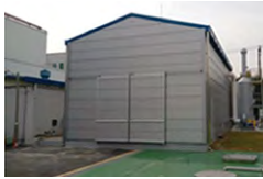
Wastewater treatment plant
