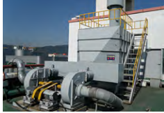
Activated carbon adsorption facility
