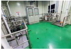
Wastewater treatment plant facility
