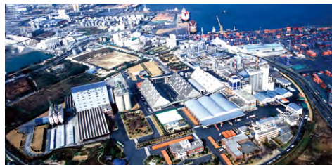
Samyang Corporation Ulsan Plant 1
