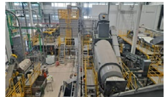
Samyang EcoTech Sihwa Plant
