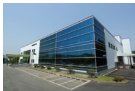
Completed construction of the Daedeok Pharmaceuticals Plant
