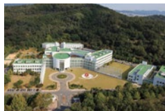
Samyang Corporation Central Research Center (Daejeon)
