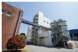
Completed construction of the Jeonju Polyester Plant
